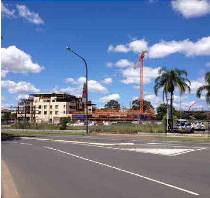
Figure 59: Looking towards the site over High Street
